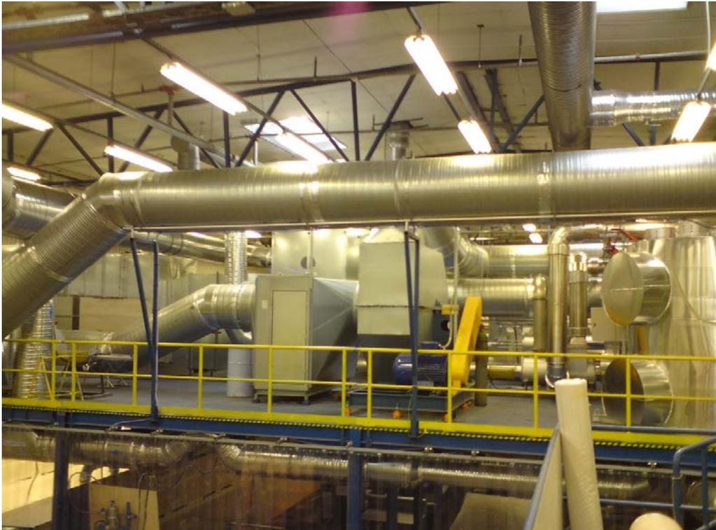
**Picture 2: Catalytic gas purification system (capacity of 40.000 m<sup>3</sup>/h)**
